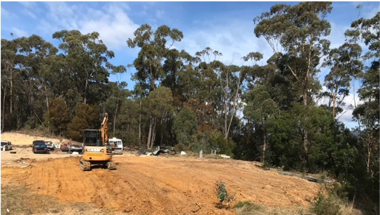
Earthworks in preparation for the new shed and carport
